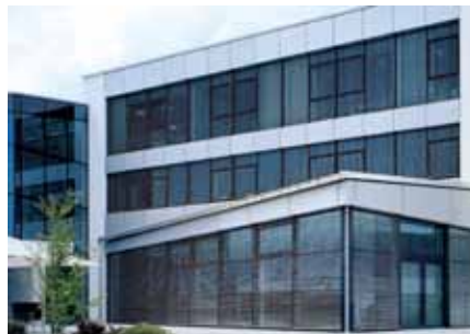
Hexal Building - Holzkirchen, Germany
