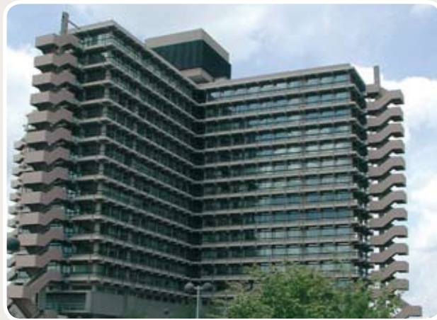
Fig. 1 South West corner of the building located in Bonn
